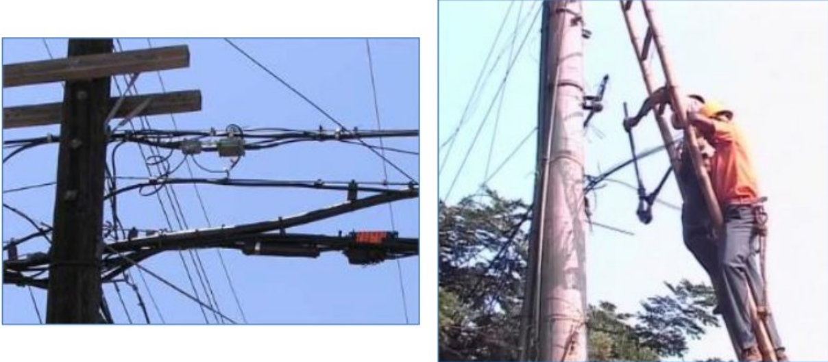
Figure-2.9 Installation of overhead fiber optic cable line
